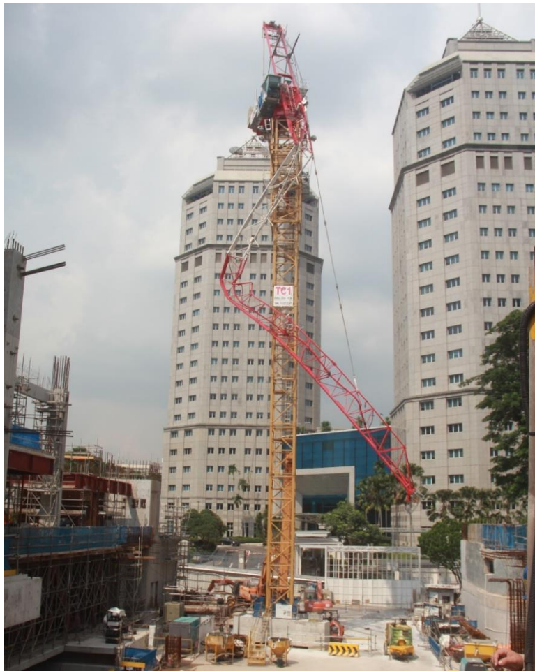
Figure 1 – General view of the TC after the accident
