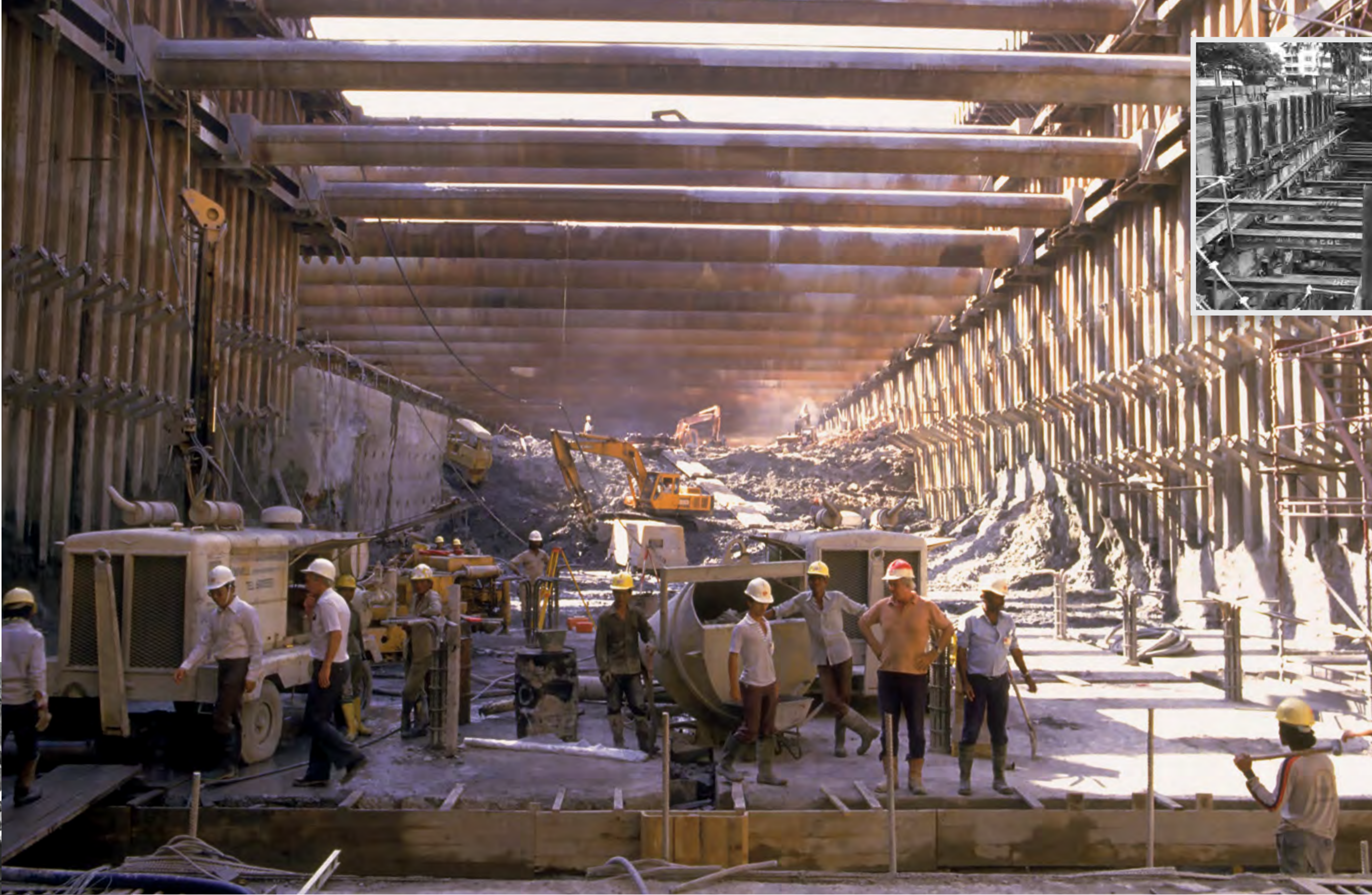
TOP: Steel beams and pillars provided the sturdy foundation for the Mass Rapid Transit tunnels.
