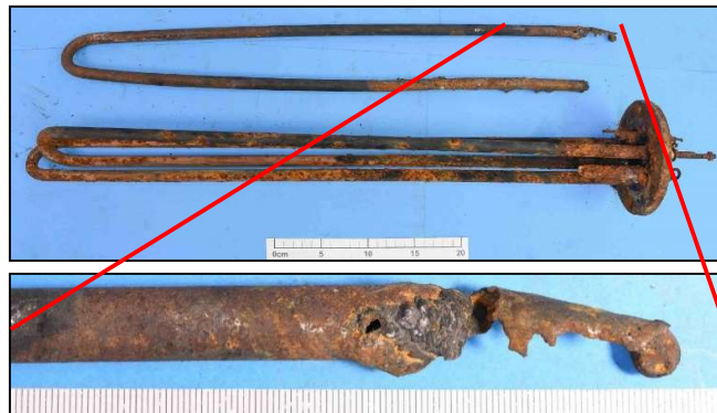
Figure 51: Post-explosion view of spoilt heater, likely to be heater #1, that was replaced on 8 August 2020
