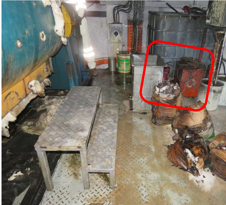
Figure 41: Welding set on platform, encircled in red
