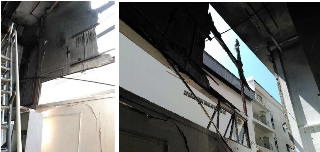
Figure 29: Photos showing dual tones on the rear back wall of the worksite
