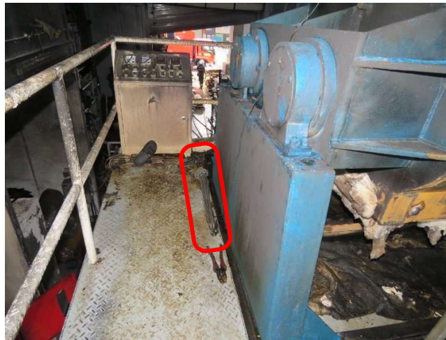
Figure 36: Heater found next to Mixer Machine, encircled in red
