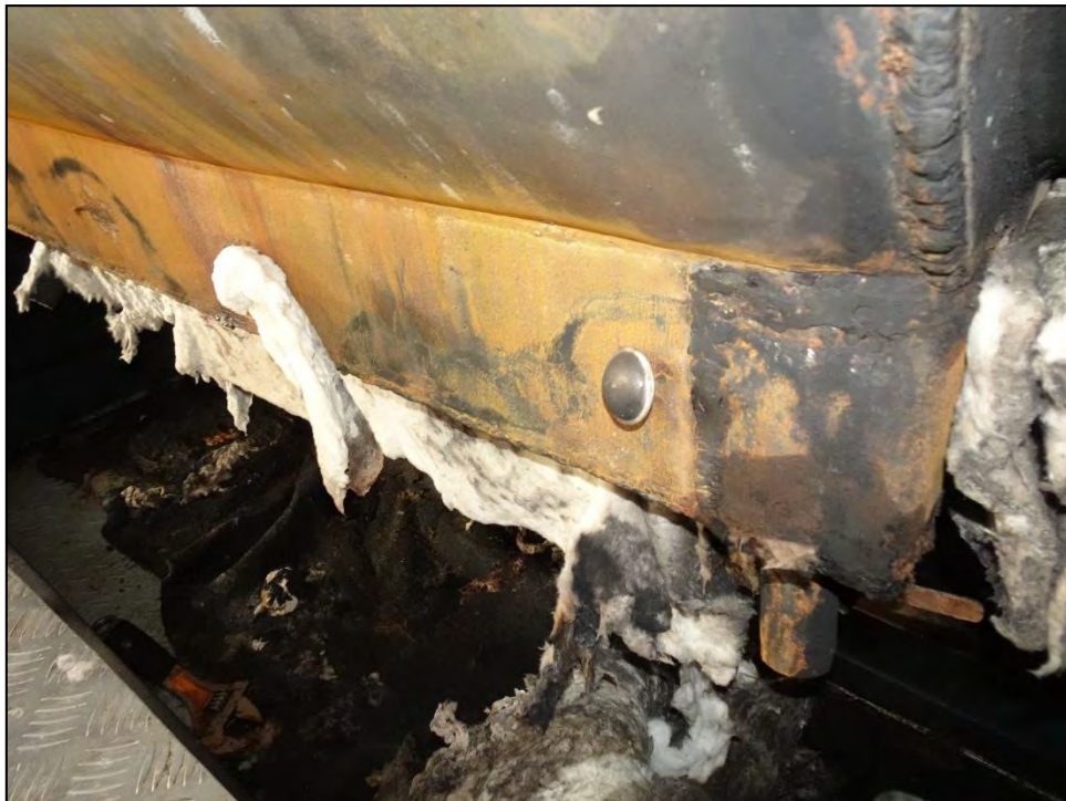
Weld repair area on the oil jacket at the front of the Mixer Machine
