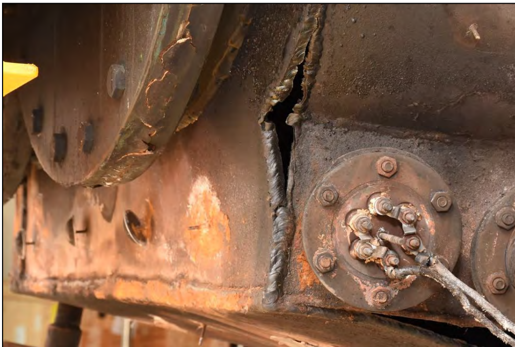
Figure 32: Close-up view of the rear left bottom corner.
