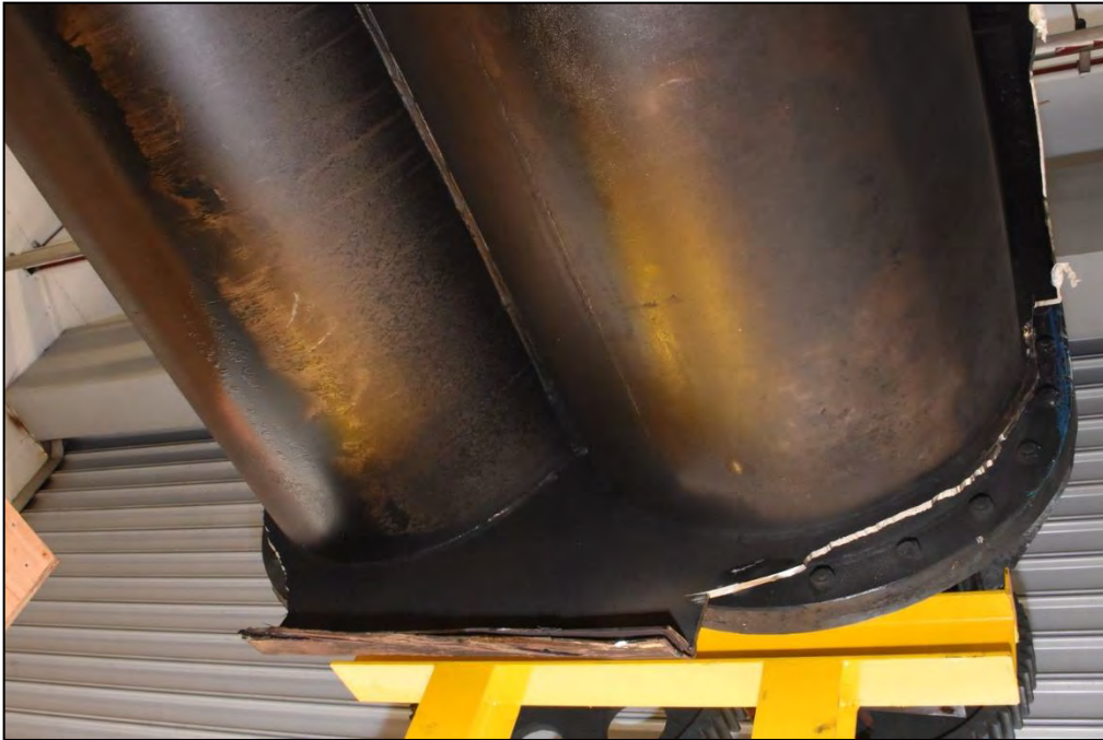
Figure 73: Internal condition of the oil jacket surface, view from the bottom showing the “W” shape of the mixing chamber formed by joining two half cylinders. Surface was generally covered with soot and oil remnant.
