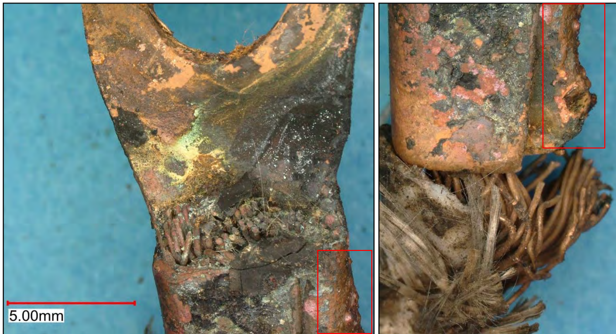
Figure 133: Condition of lug before cleaning.
