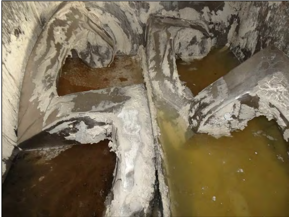
Internal condition of mixing tank
