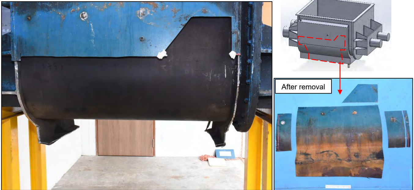
Figure 39: Internal condition of the oil jacket from the front side. The internal surface was generally covered by black soot.
