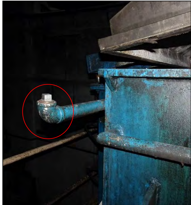
Access port to top up oil (circled, left) and vent port of oil jacket at the rear side (circled, right)
