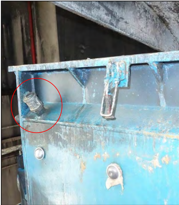
Access port to top up oil (circled, left) and vent port of oil jacket at the rear side (circled, right)
