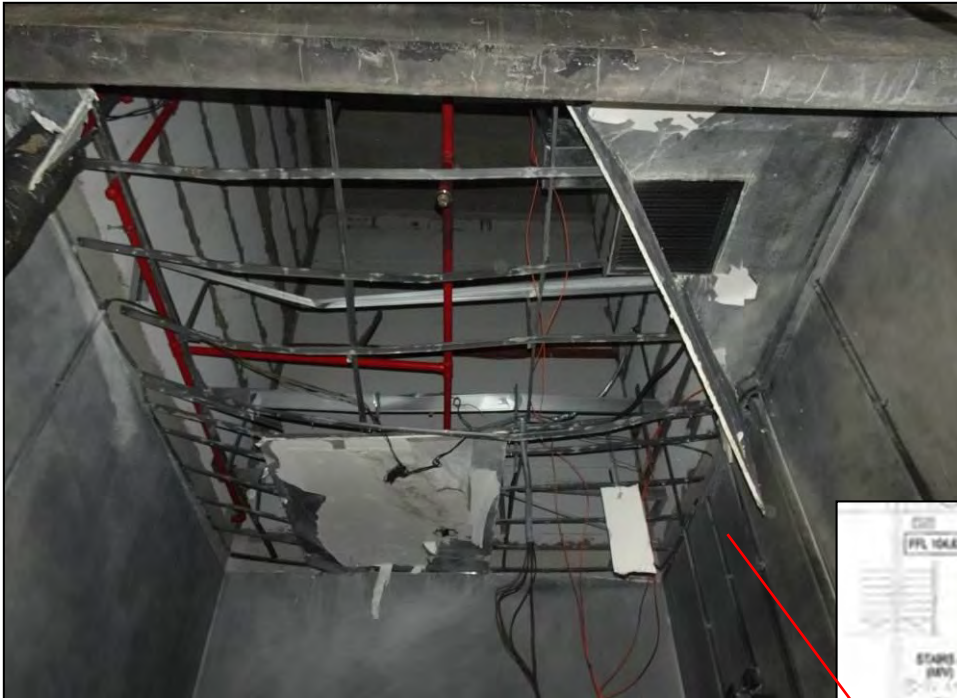
Top of the area near the lift
