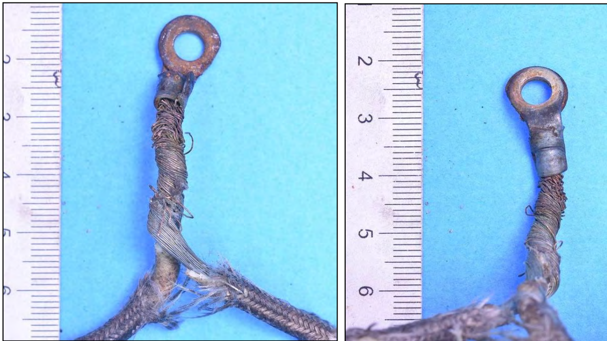
Figure 132: Wire and lug of heater #2, terminal 4.
