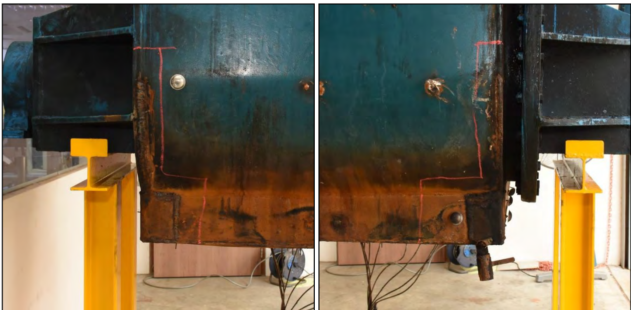
Figure 38: Marked out locations on the front corners for detailed examination.
