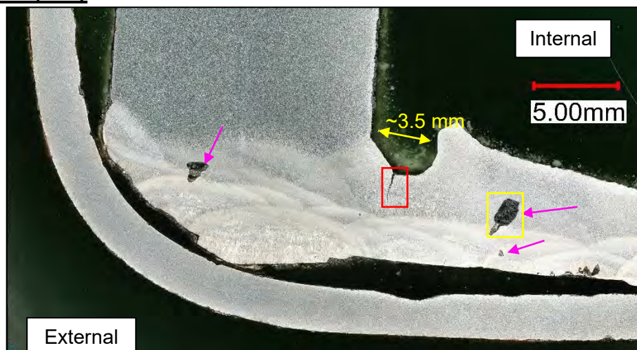
Figure 155: Sectional metallographic examination was conducted across the repair weld and corner reinforcement plate. Lack of root penetration was observed with a root opening of about 3.5 mm wide. Voids of up to 2.5 mm wide were scattered in the weld metal (in pink).
